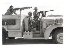
A 'T1' Patrol Chevrolet 1533X2 30 cwt: the small drum behind the fender is the <u>radiator condenser</u> and the truck's sand channels are mounted on brackets on the rear bodywork. The weapons are the <u>Lewis gun</u> (left) and a .303 Browning Mk II (right)
